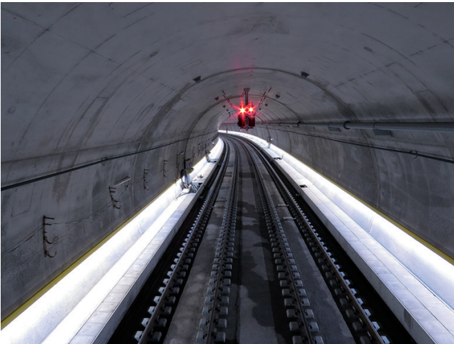
Overall view of SBB-cross city link Zurich
