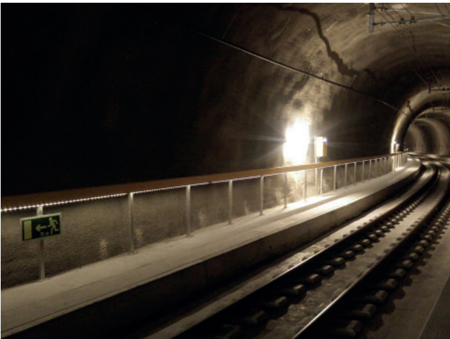
Installation tunnel Ruckhalde Appenzeller Bahnen
